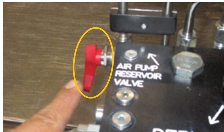
Figure 5.16 - Air Pump Reservoir Valve (Isolator Valve) - Shown in Open Position
